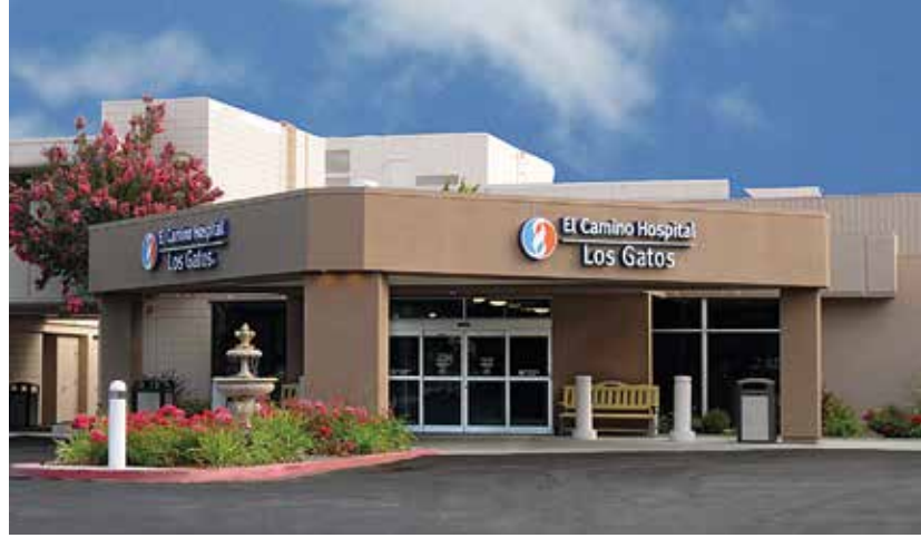
El Camino Hospital, Mountain View
